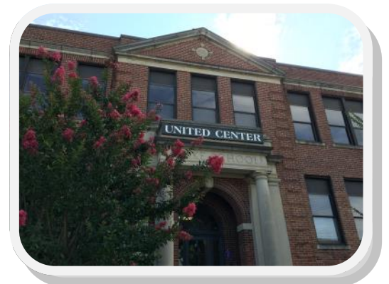
New Location for the LLLN Office
